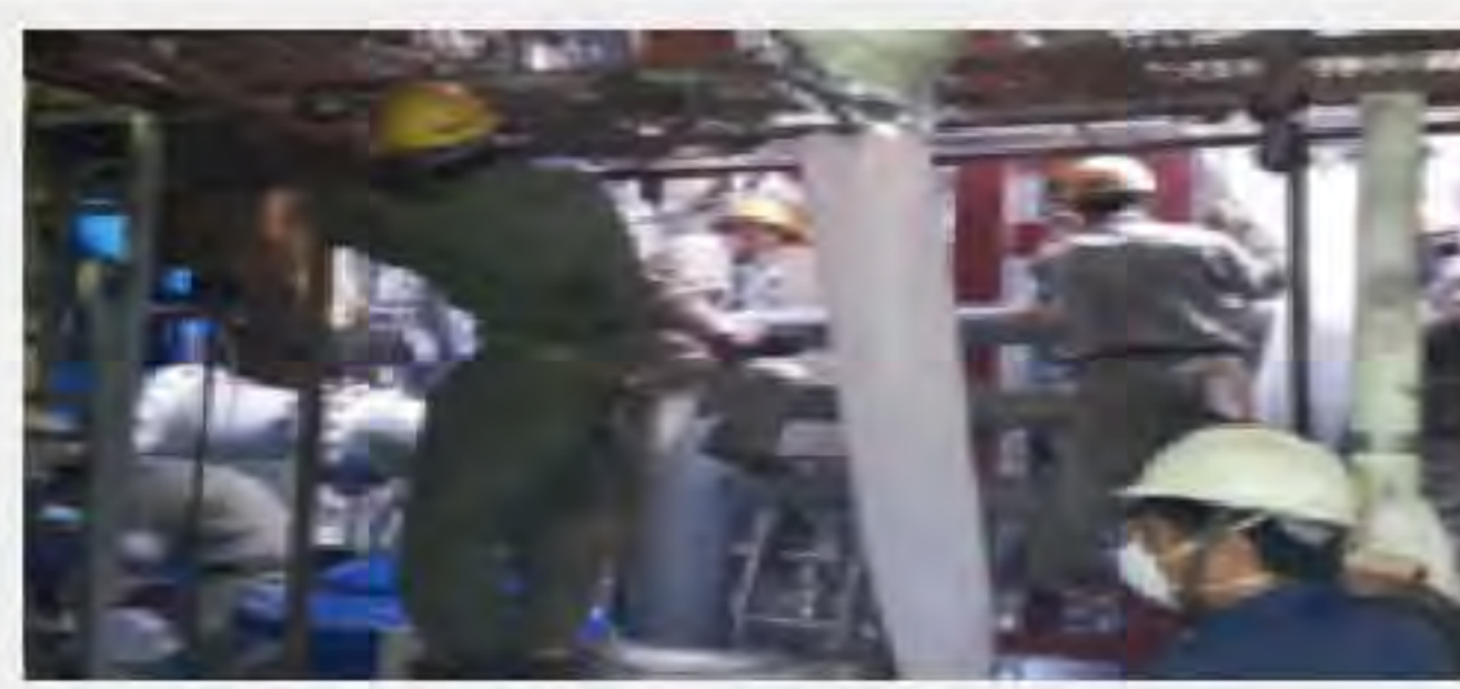
Supervision During Prefabrication, Installation and Commissioning
