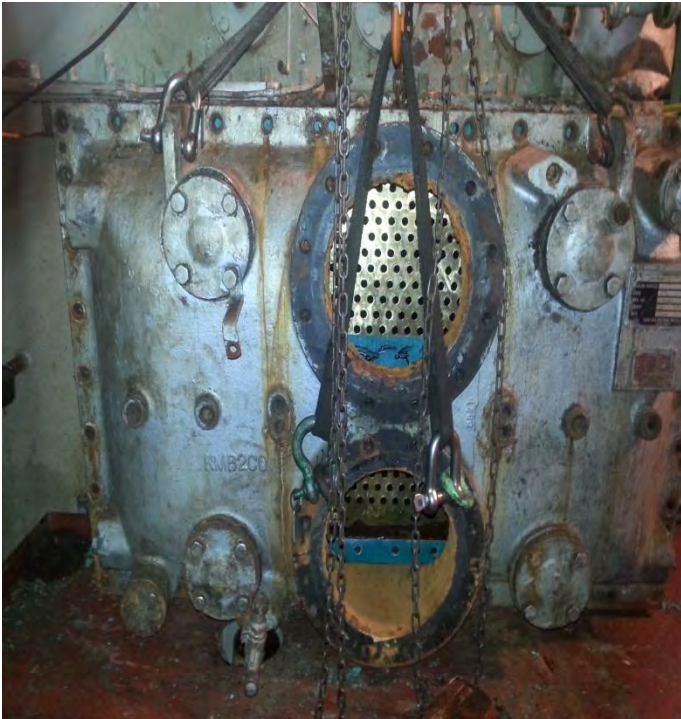
Existing Marine Engine of Air cooler removed from on board
