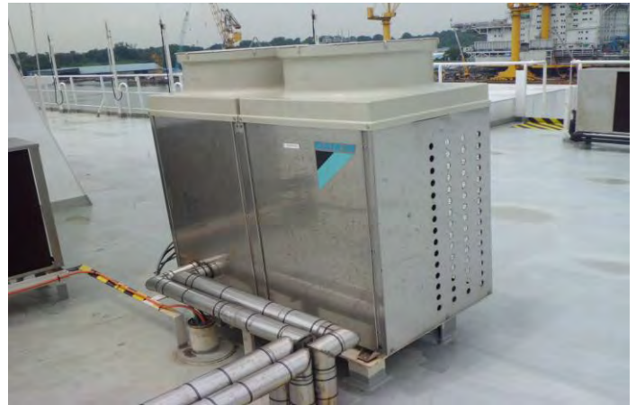
Assembling of Chiller Unit
