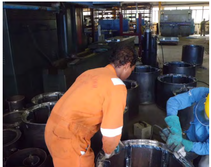
Steel work in Progress
