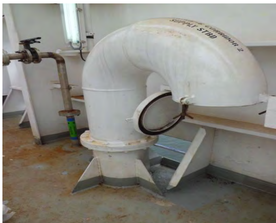
Fabrication & Installation of Gooseneck
