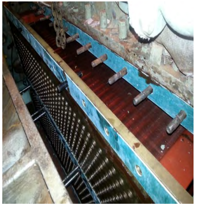
New Marine Engine of Aircooler Installation
