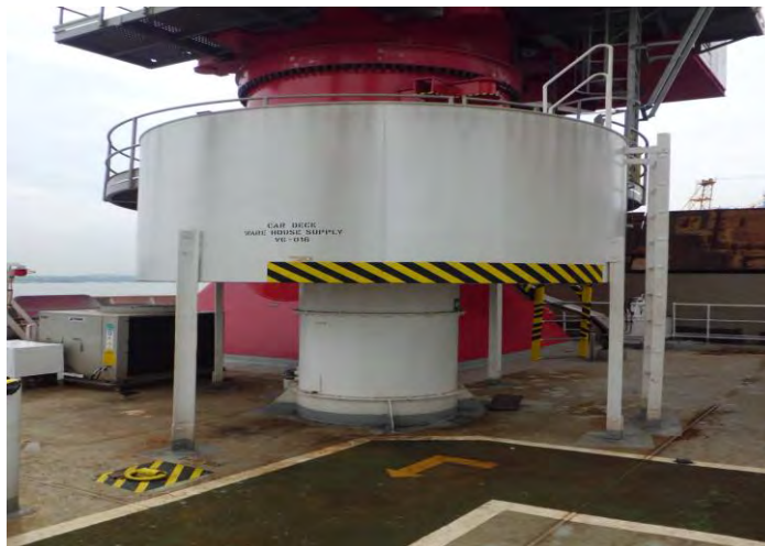
Installation of Mushroom on-board
