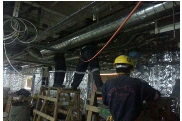
Installation of spiral ducting
