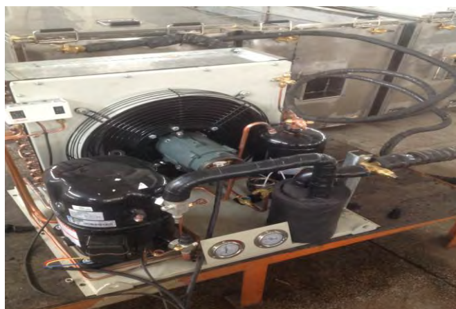
Reconditioning of Compressors
