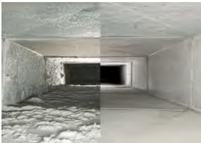
Ducting cleaning before and after
