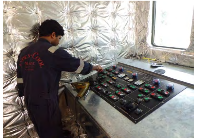
Installation of Control Panel switch
