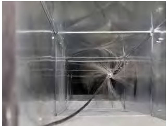
Duct cleaning Final Inspection
