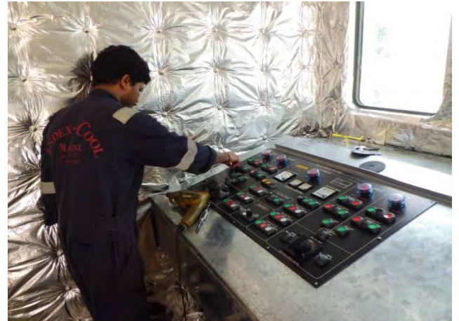
Installation of Control Panel switch
