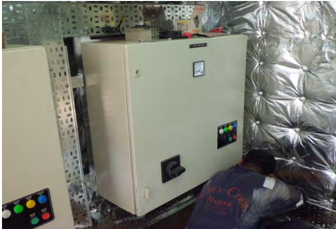
Installation of New Control Panel
