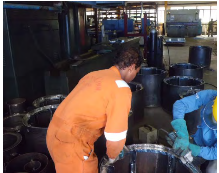
Steel work in Progress
