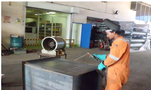
Fabrication of New Trunking in Progress
