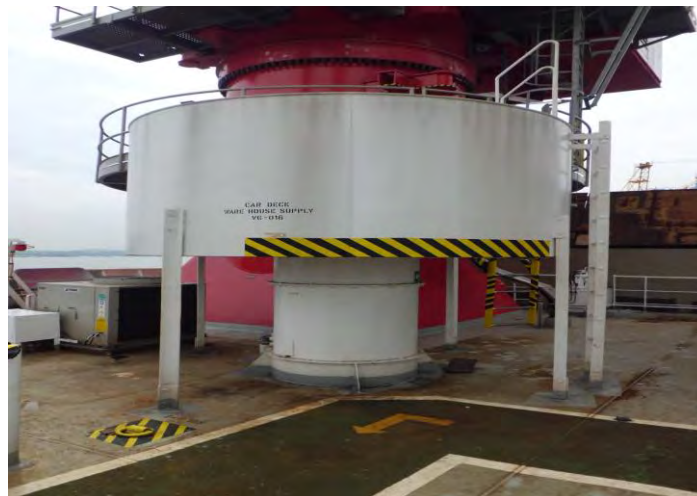
Installation of Mushroom on-board
