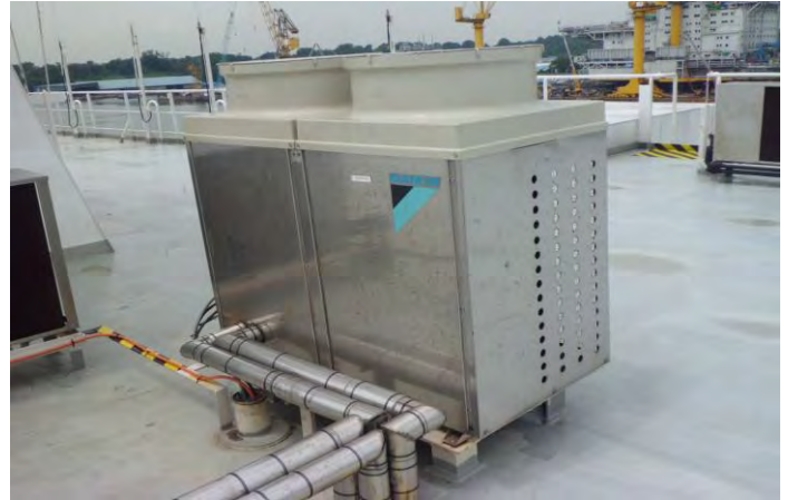
Assembling of Chiller Unit
