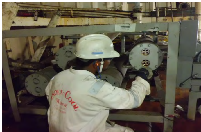
Assembling of New Condenser
