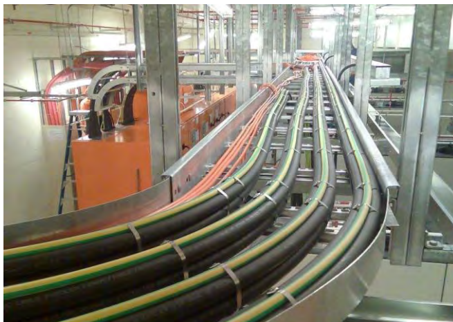
Laying of cable on board
