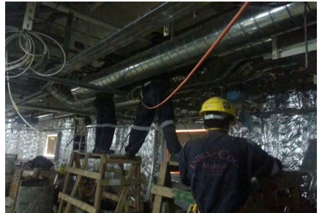
Installation of spiral ducting
