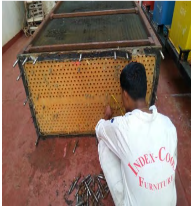
Existing Marine Engine of Air Cooler Measuring Dimension
