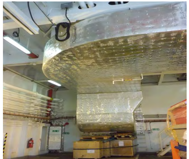
A60 Insulation on board
