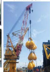
Vessel Crane Load Testing
