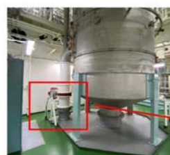
IG Scrubber SW line ND 400 (existing pipe)
